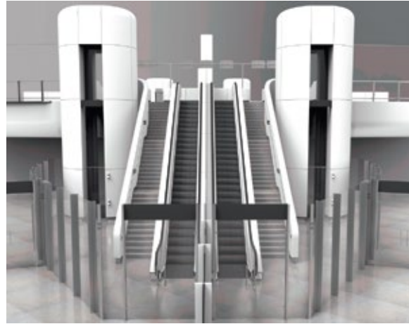
Figure 19 - Elevators and escalators view from the PTB
