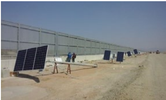
Figure 5 - Erection of luminaires North Junction
